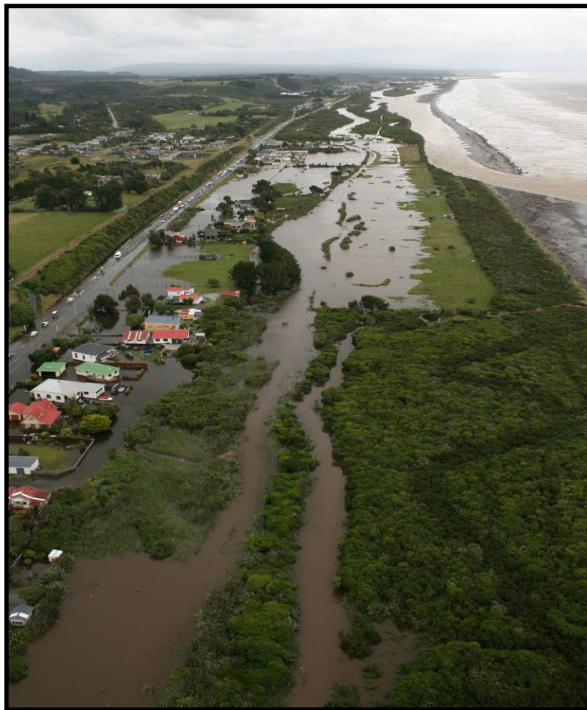
Flooding at Saltwater Creek, Paroa, 28 December 2010 photo courtesy of Jason Boddy
