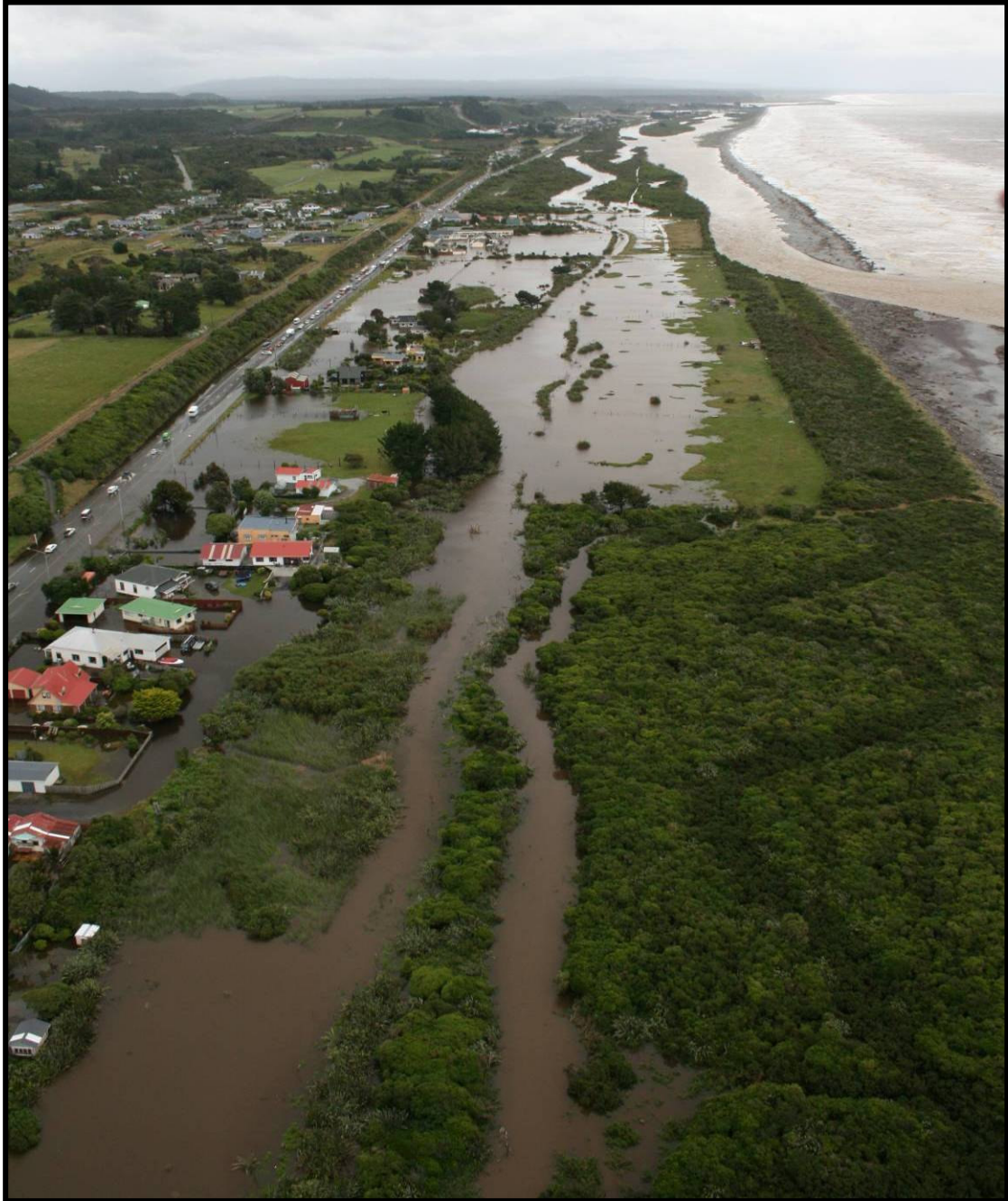
Photo showing extensive flooding caused by backing up of water in the drain system north of Saltwater Creek, and the dominant flow of New River, photo courtesy of Jason Boddy
